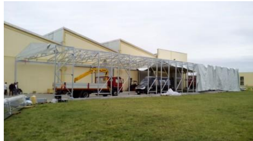
Tunnel mobile (BOLOGNA)
