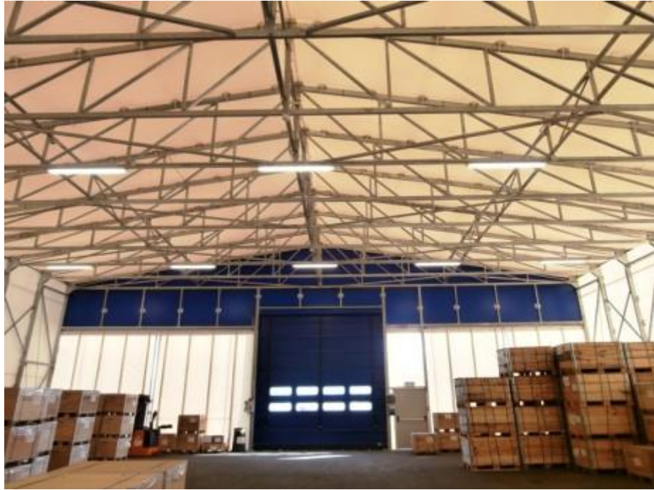
C.M. – COPERTURA MOBILE TUNNEL HANGAR (VICENZA)
