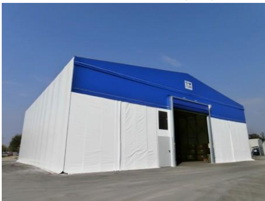
C.M. – COPERTURA MOBILE TUNNEL HANGAR (VICENZA)
