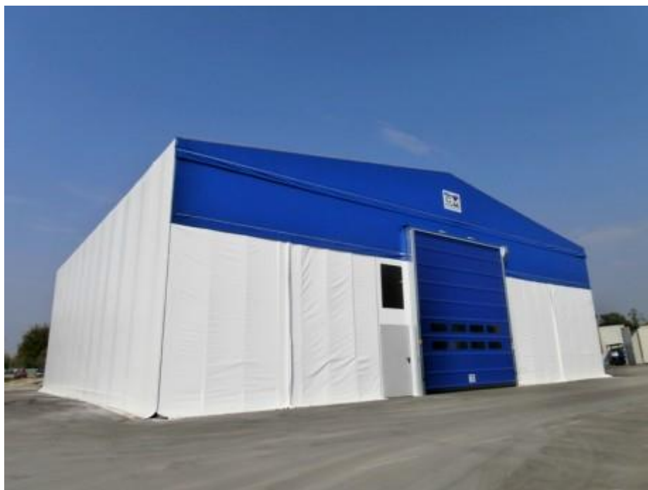
C.M. – COPERTURA MOBILE TUNNEL HANGAR (VICENZA)
