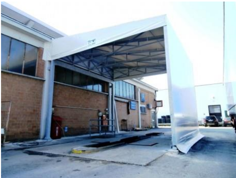
C.M. TETTOIA TUNNEL MOBILE (REGGIO EMILIA)
