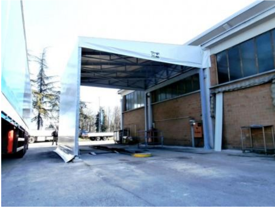
C.M. TETTOIA TUNNEL MOBILE (REGGIO EMILIA)
